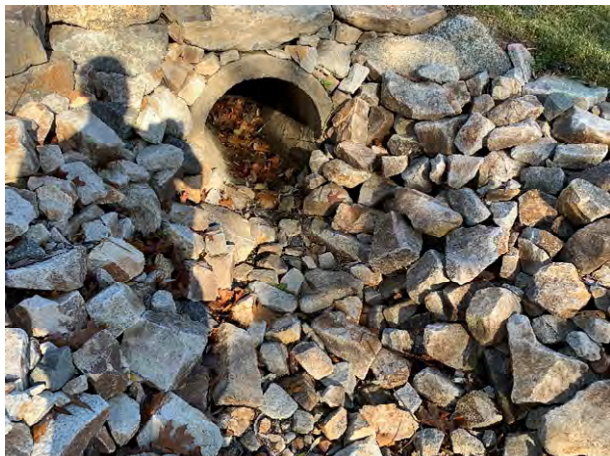
64 Gundalow - 1 (Drainage Course)
