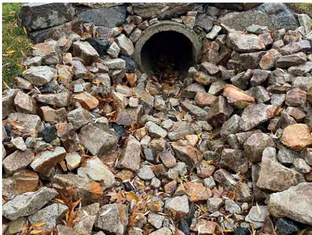
64 Gundalow - 1 (Drainage Course)
