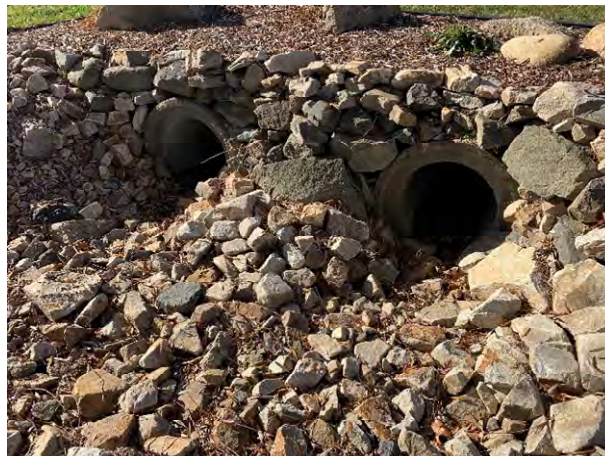
64 Gundalow - 2 (Drainage Course)
