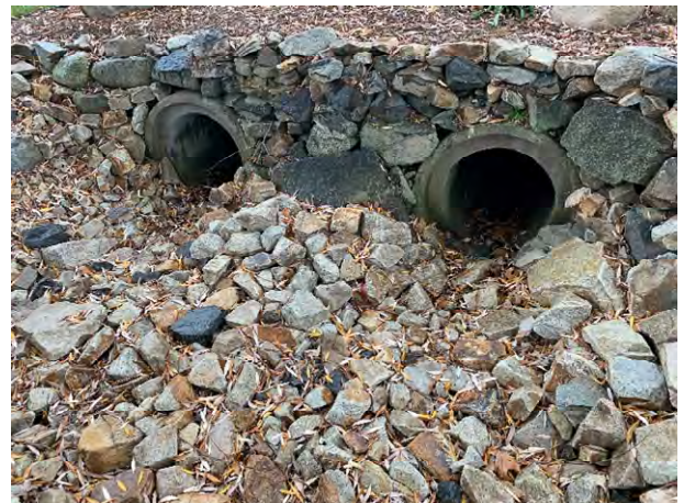
64 Gundalow - 2 (Drainage Course)
