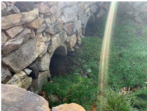
4 Brickyard Circle - 1 (Drainage Course)
