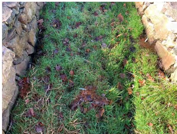
4 Brickyard Circle - 2 (Drainage Course)
