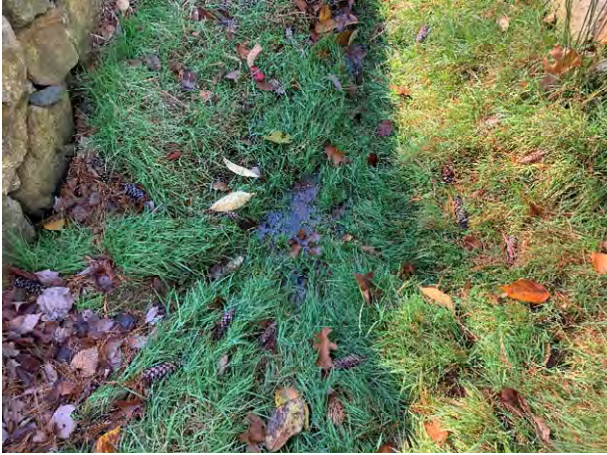
4 Brickyard Circle – 3 (Drainage Area)
