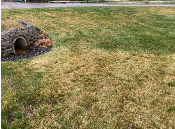
29 Gundalow - 1 (Drainage Area)
