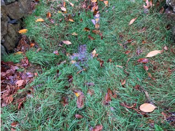
4 Brickyard Circle – 3 (Drainage Course)
