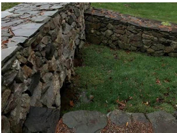
4 Brickyard Circle - 1 (Drainage Course)
