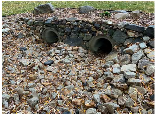
64 Gundalow - 2 (Drainage Course)
