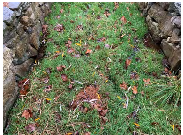
4 Brickyard Circle - 2 (Drainage Course)
