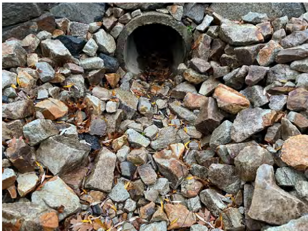
64 Gundalow - 1 (Drainage Course)
