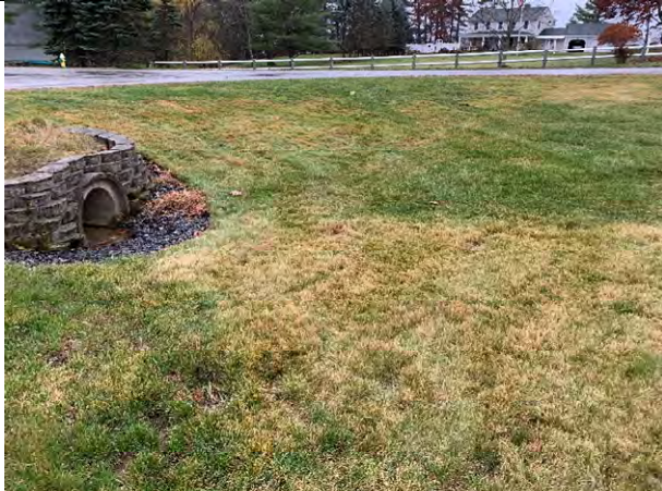
29 Gundalow - 1 (Drainage Area)
