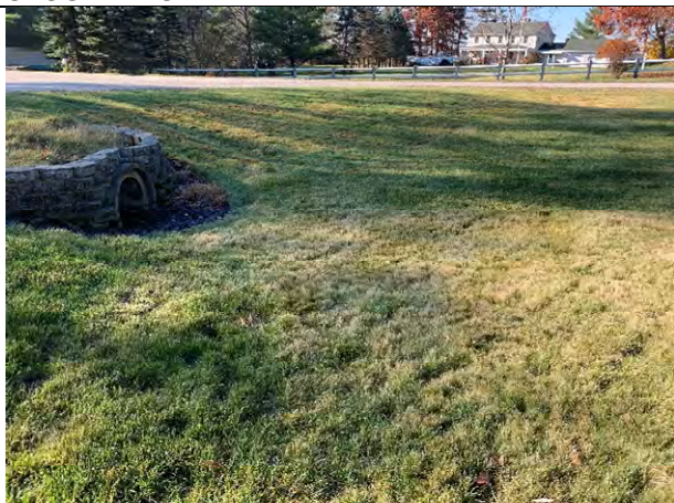
29 Gundalow - 1 (Drainage Area)
