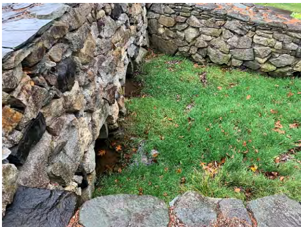
4 Brickyard Circle - 1 (Drainage Course)
